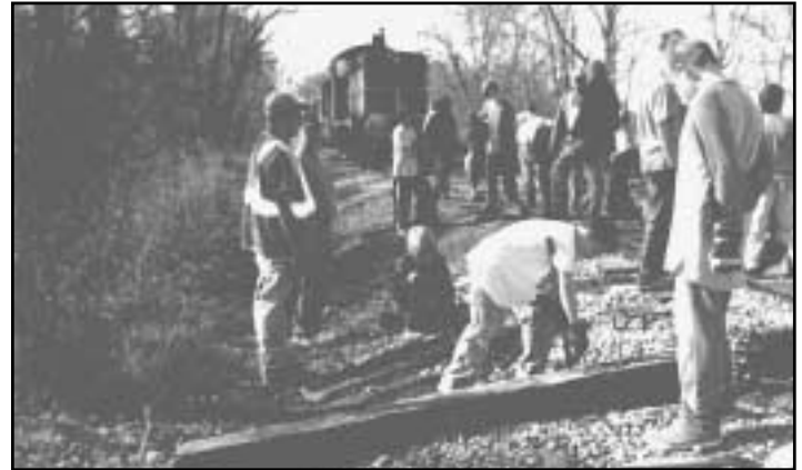
MEMBER BLAIR ADAMS supervises Boy Scouts during Nov. 17, 2009 Train Camp. Here, boys are "plugging" a crosstie, making it ready to slip under the rails and be spiked into place.
